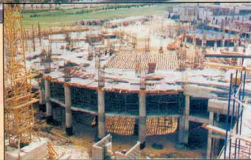
CCC/Orascom are building the Marriott Mirage Hotel
